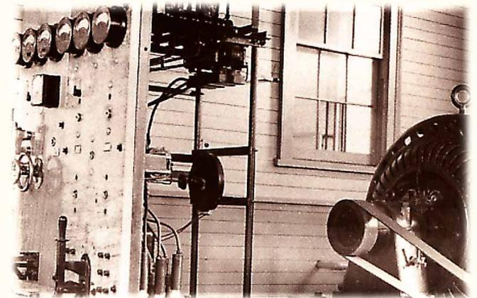
*In 1940 a 50 kilowatt diesel unit was installed at St. Quentin*
