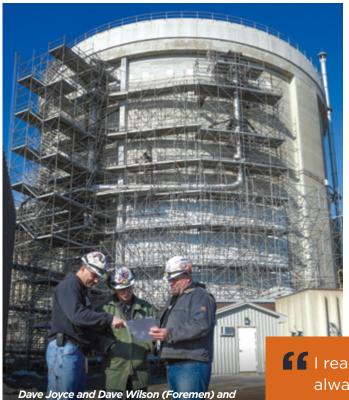
reliably. There is a total of 13,851 scaffold pipe pieces that highly trained and qualified scaffolders and carpenters installed on the outside of the reactor building, which are equal to 67,974 linear feet of scaffolding material.
