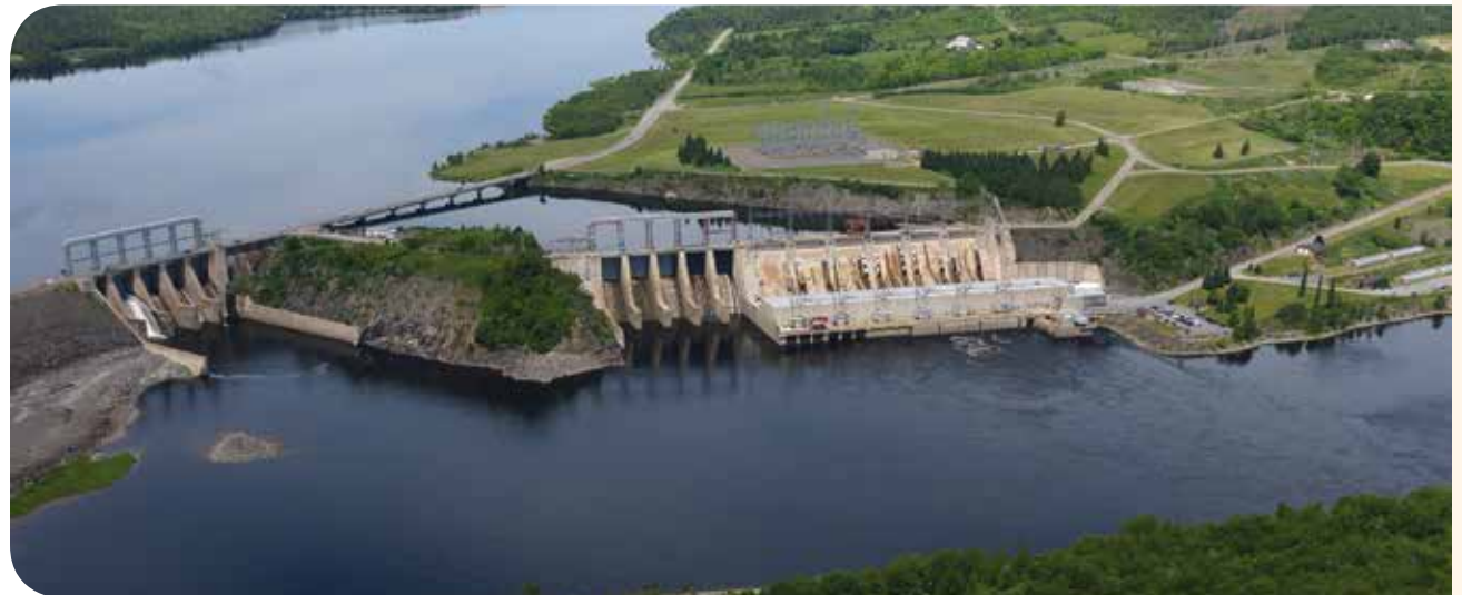
Mactaquac Generating Station
