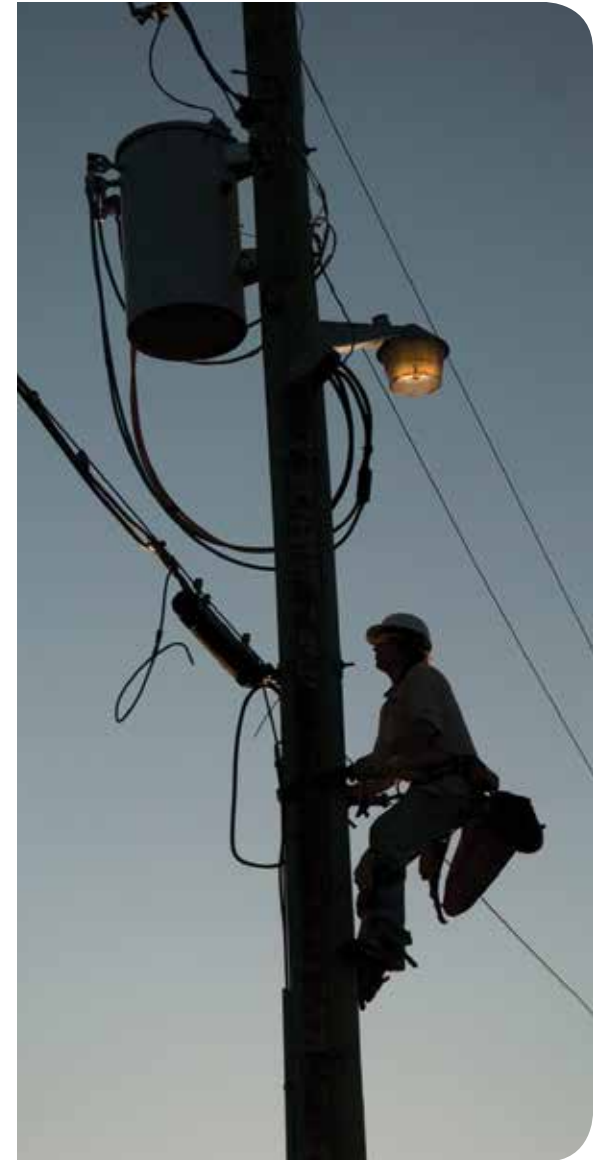
Lineman working in Bathurst, NB.
